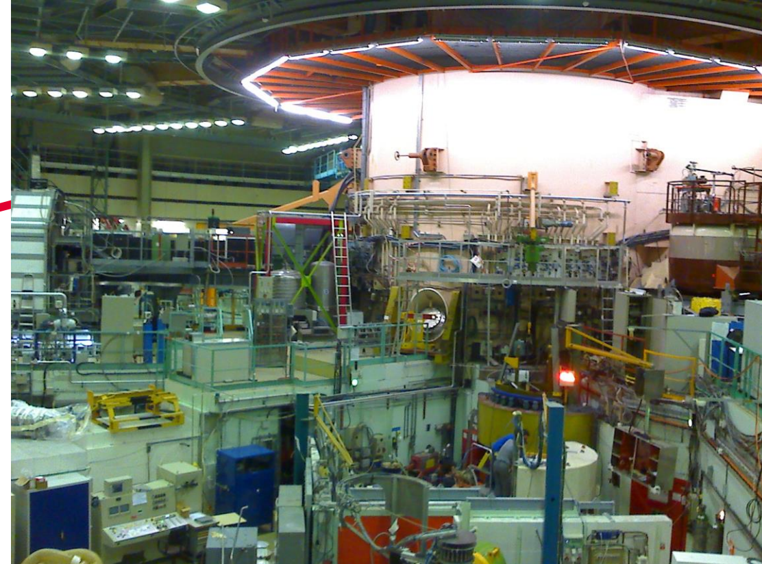
Inside the reactor hall
